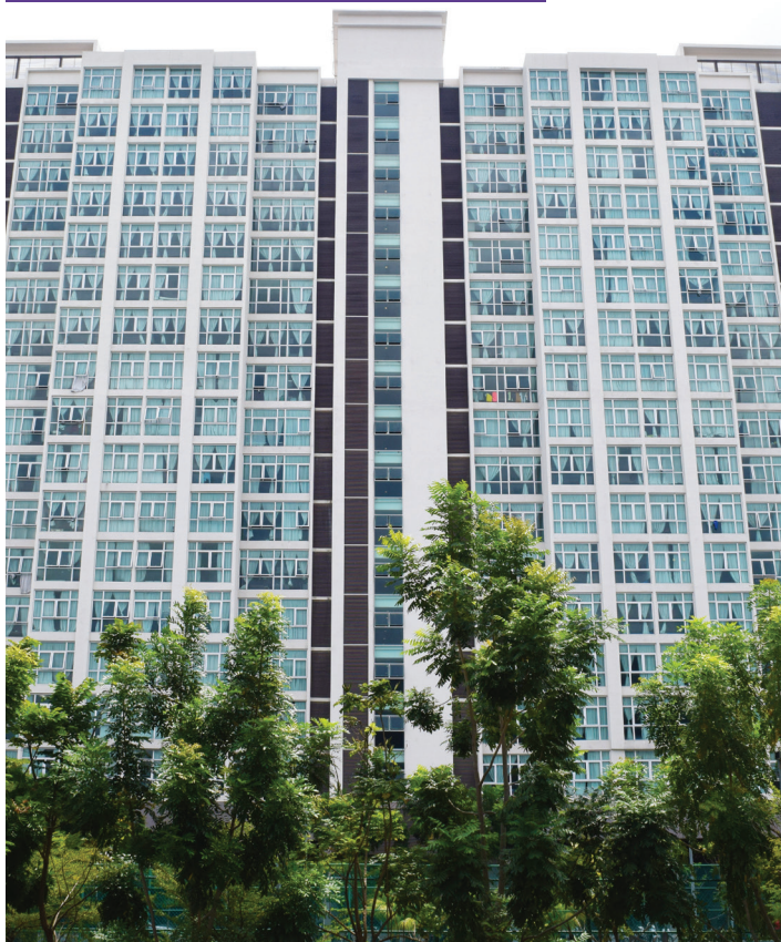
Front View of Seri Mutiara Hostel
